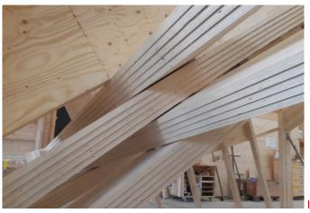
The beams are made of spruce laminated veneer lumber and arranged as a lattice shell. In total, 20 kilometres of LVL panel strips make up the grid of the roof support structure.
