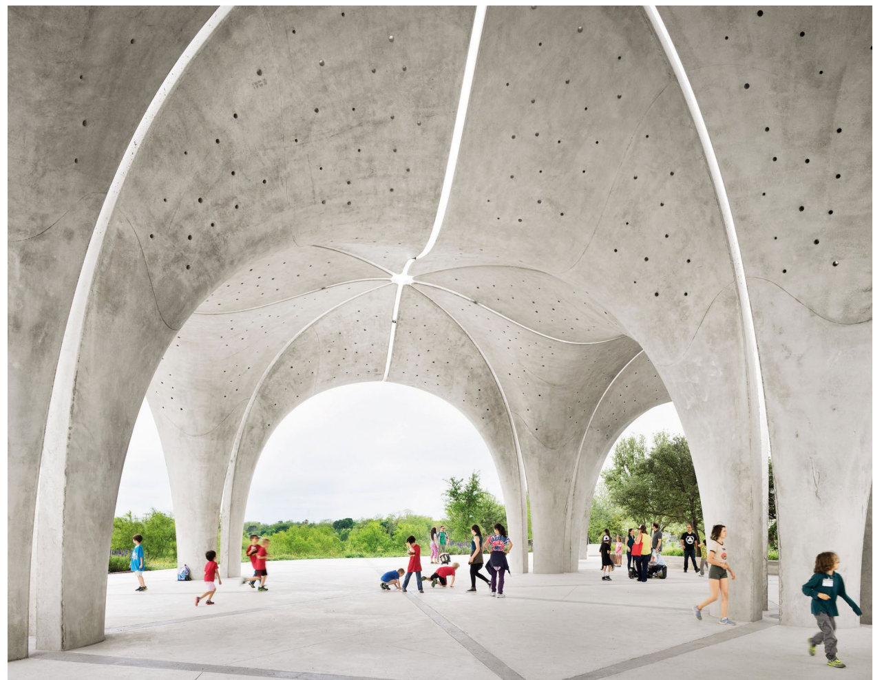
1. Aerial view of Confluence Park showing the smooth fibreglass finish and broom-finished concrete surfaces. The namesake of the park, the confluence of the San Antonio River and San Pedro Creek, is shown in the background. Credit: Rialto Studio.
