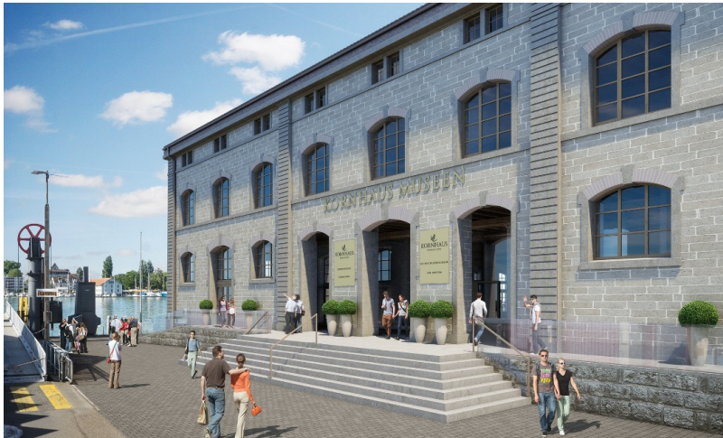
Historical structure next to the water
