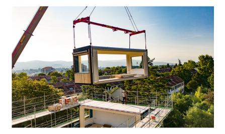
The prefabrication of the timber modules took six days. On the construction site, they were then put in place on the roof of the school building.
