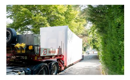
The individual timber modules were prefabricated at our factory in Gossau and then transported by low loader to the construction site.
