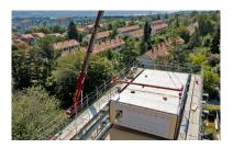
Some of the prefabricated timber modules are already in place on the roof of the primary school pavilion.
