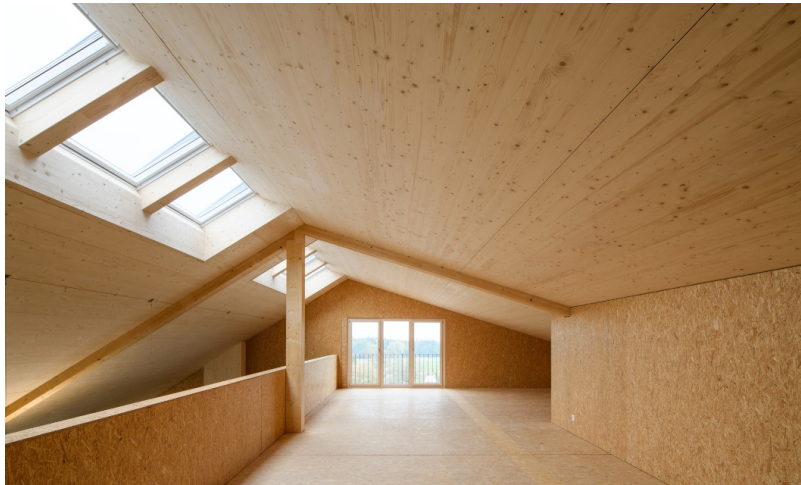
Spruce roof truss
