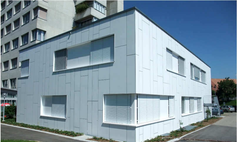
Two-storey temporary structure
